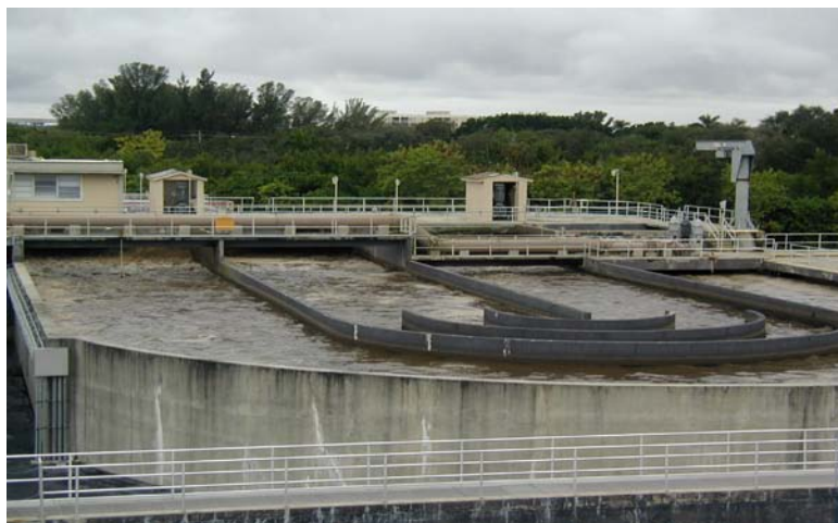
This 2.5 million gallon aeration tank which is the heart of the BardenPho process contains 83,500 pounds of micro-organisms.
