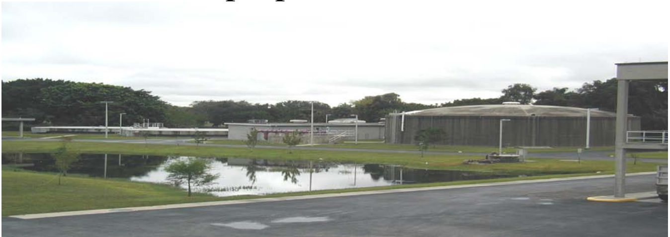
Reclaimed Water Production Facility
