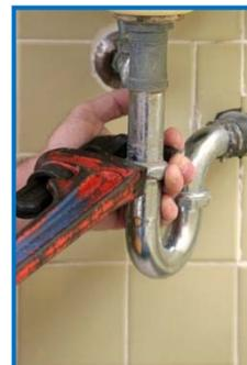
When plumbing parts are removed or cleaned, caution should be taken to avoid spilling the contents in case amalgam or mercury is present. Pour and brush out the sludge and handle it as if it were contact amalgam, or have it discarded as hazardous waste. Contact an amalgam or mercury recycler or a licensed hazardous waste handler (Appendix A) for further clarification. The plumbing parts can then be put back in place or recycled.
